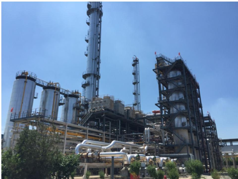
PHOTO CAPTION: Albemarle's zeolite-based AlkyStar™ catalyst has successfully produced high-quality alkylate at the world's first solid acid alkylation unit in Shandong, China. Photo provided by Shandong Wonfull Petrochemical Group Co., Ltd.
